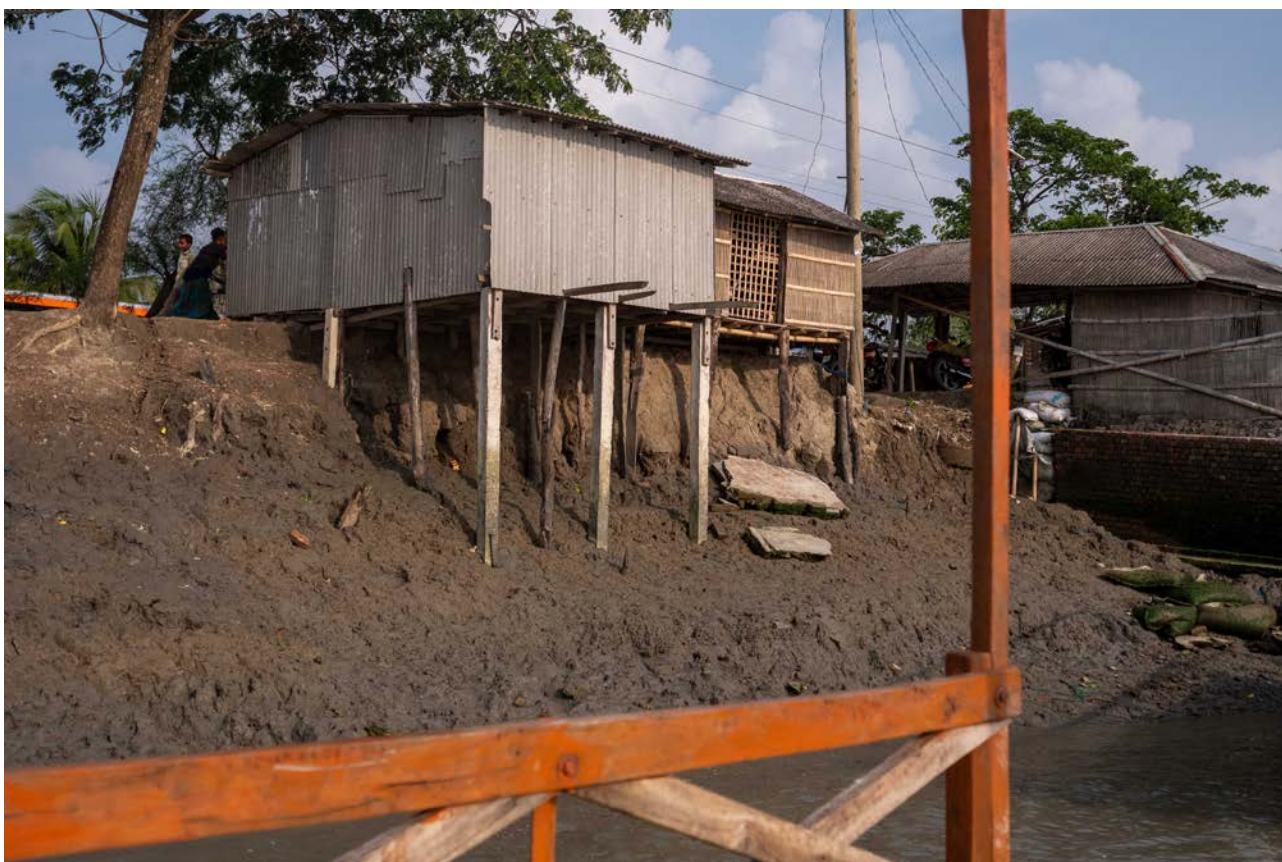
Photo 3: Riverbank erosion in Gabura Union (Credit: Douwe van Schie)
