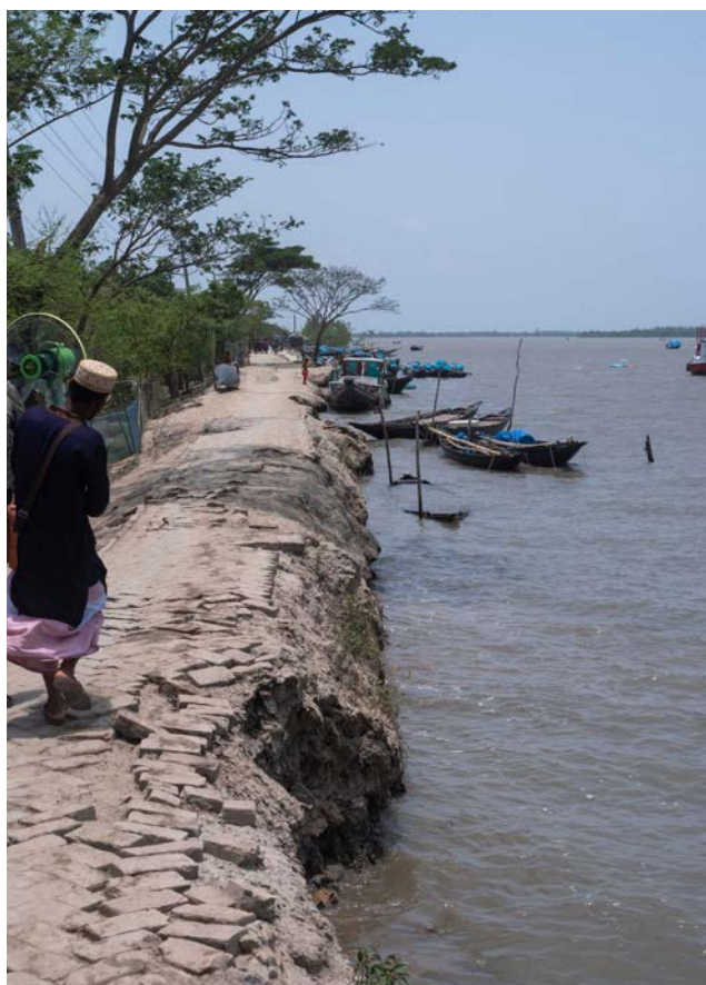
Photo 5: An embankment road in Gabura Union (Credit: Douwe van Schie)
